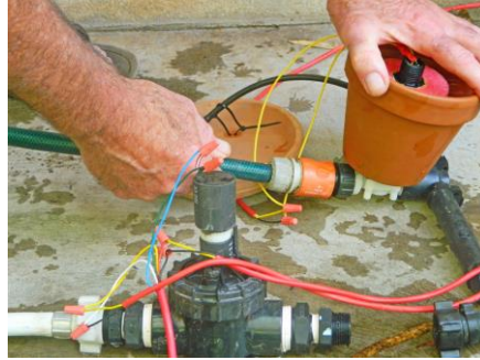
Connect the water supply to the inlet of the controller
