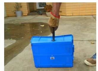
Push the pipe through the grommet
