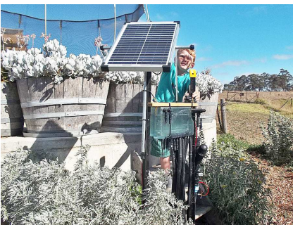
Sophie's son Beau adjusts the angle of the 20 watt solar panel.
