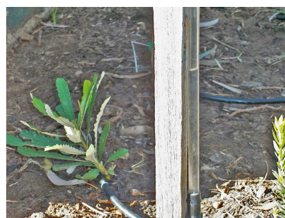
Pressure monitor tube indicating the water pressure in the zone
