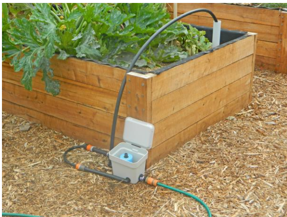
Installation of Unpowered Wicking Bed Controller
